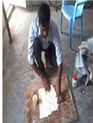
Applying polyester sheet
